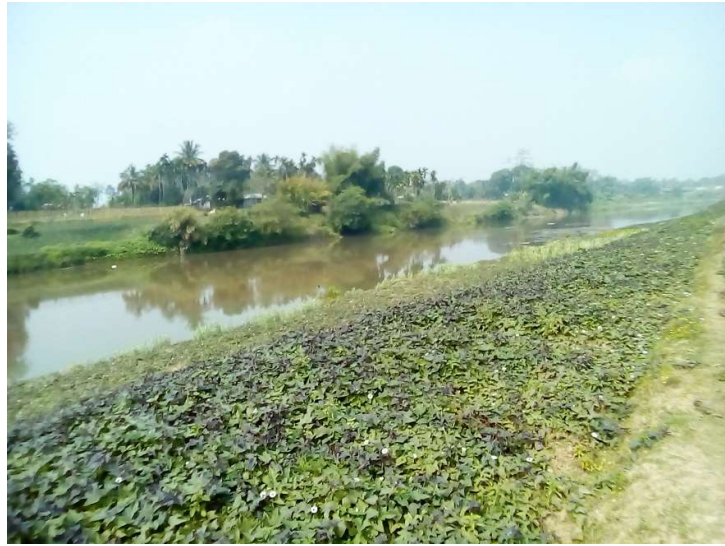
Figure 2:Current Status of the Project Site
